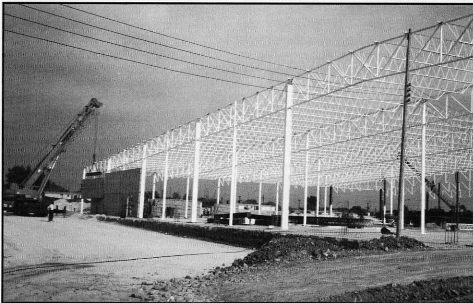
Pre-cast concrete panels are added to the structural steel of Guadalupe I.
