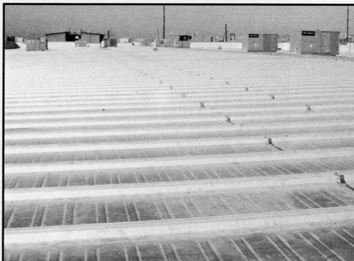
The latest roof system — a standing seam metal system — is used in all new construction.
