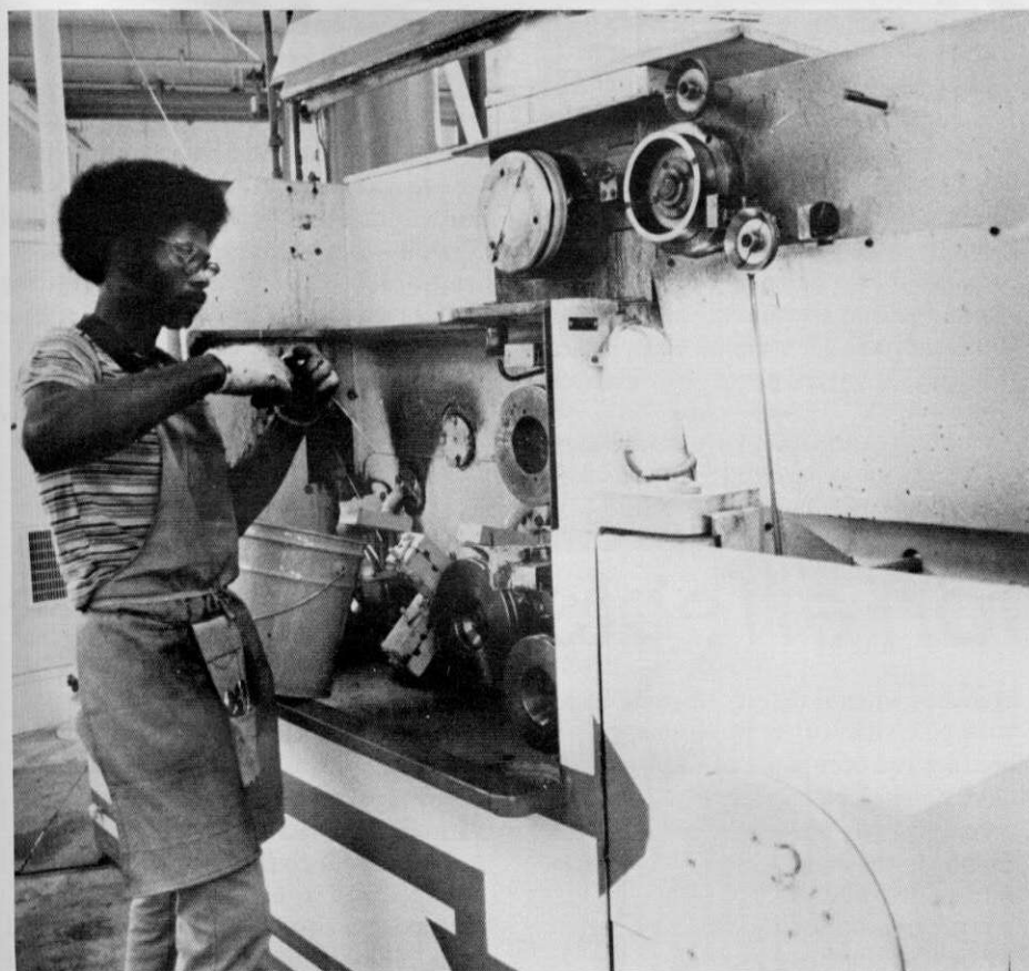
ROBERT MILTON , Dept. 2234 rod mill operator, checks wire drawn through one of the machines he operates in the High Speed Cable Module.
